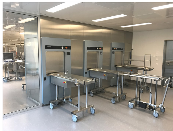
New ZSVA in the canton of Argau: RGD & sterilisers
